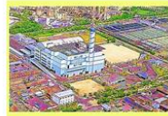
KOGASAKI INCINERATION FACILITY City of Kitakyushu
